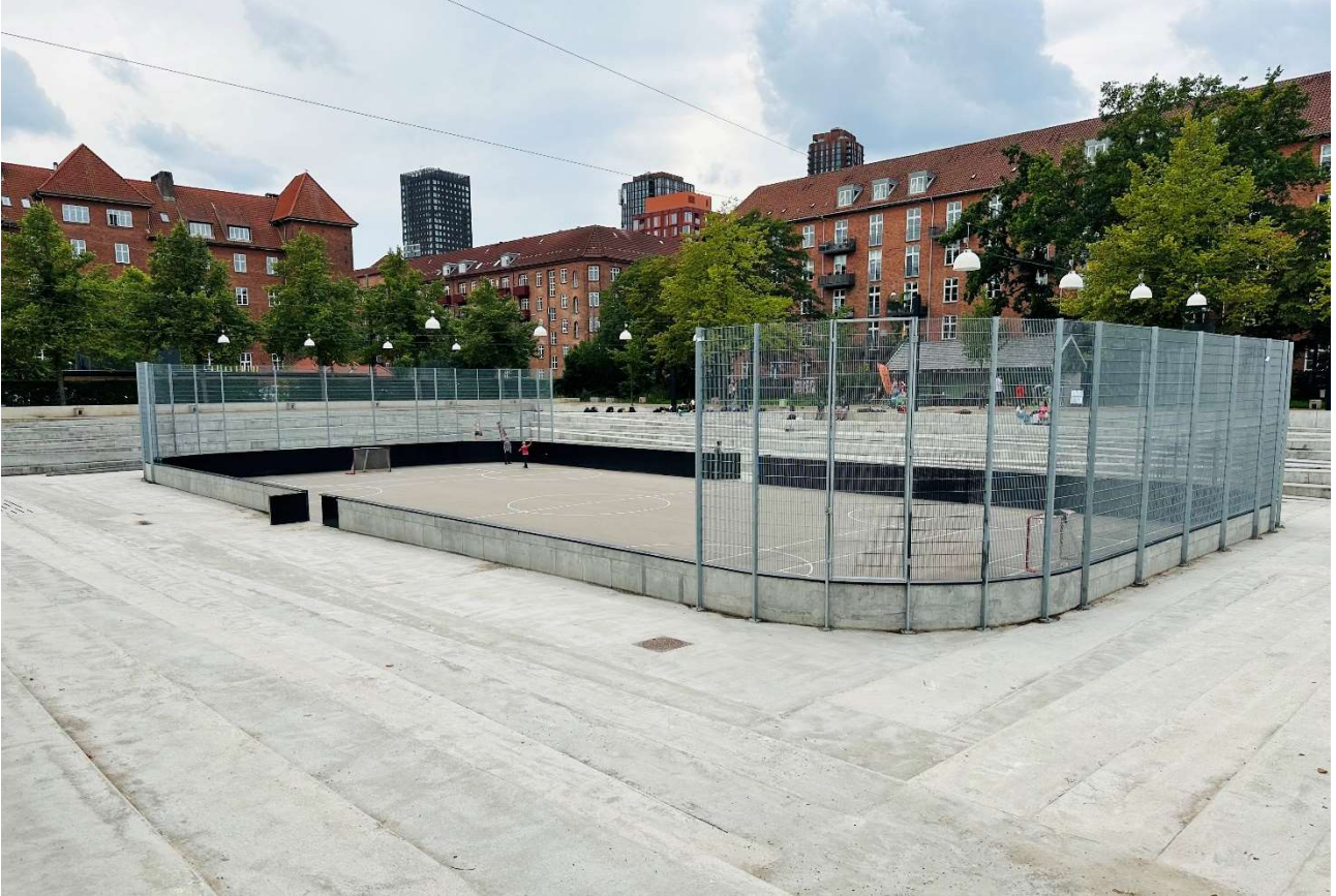
Figure 6: Sunken multi sports 'court' designed to temporarily store flood water as part of Enghaveparken, Copenhagen
