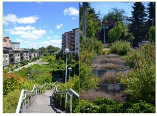
Stormwater management in Seattle. Daylighted Thornton Creek through development (left) and retrofitted raingardens at 101 Cascades (right)
